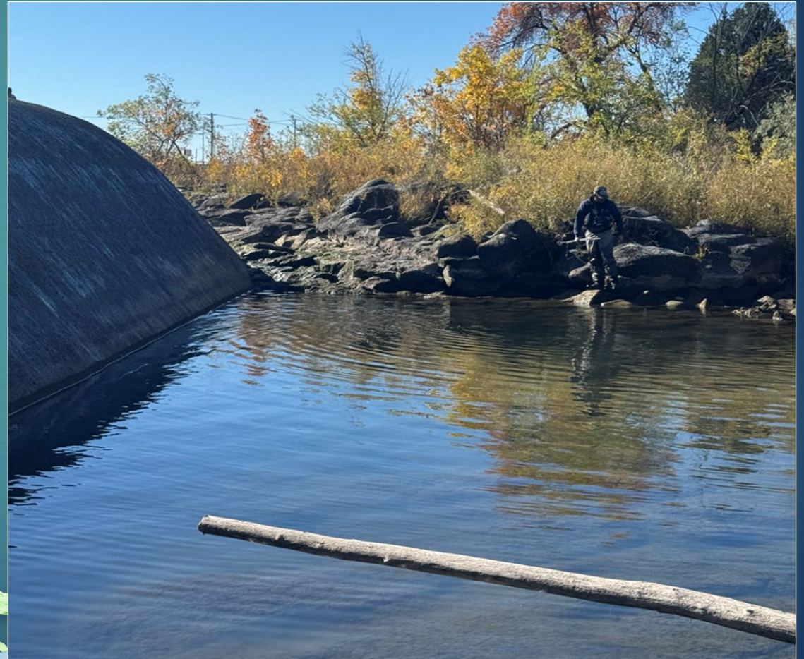
↓ Left channel plunge pool below spillway
